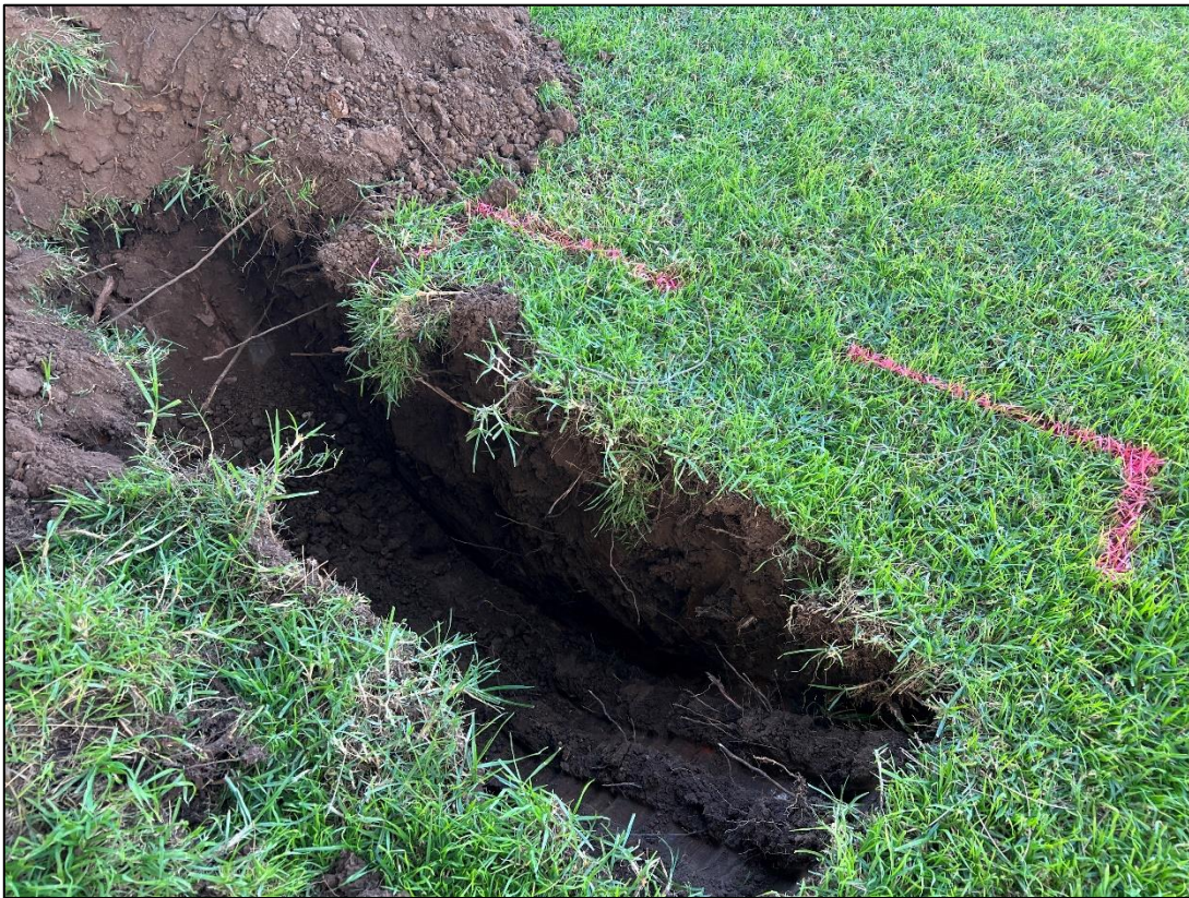
Image 26: Test pit TP10 (taken 13/04/2023)
