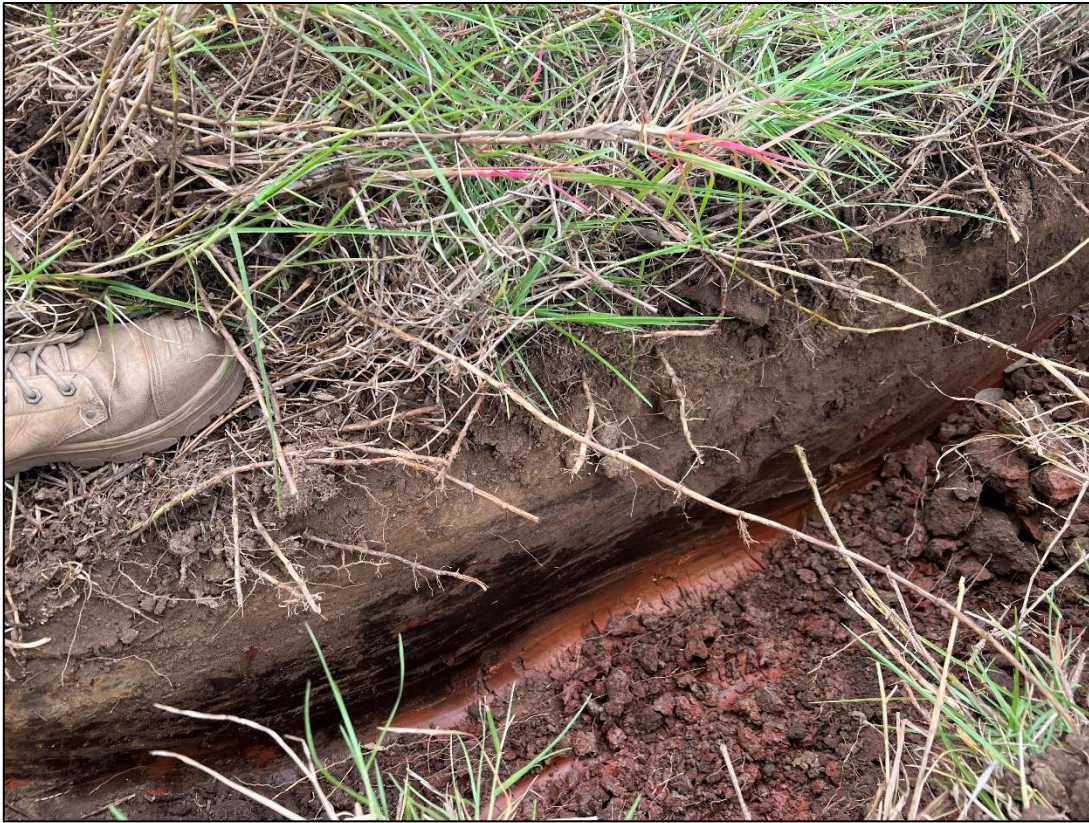
Image 15: Test pit TP01 (taken 13/04/2023)
