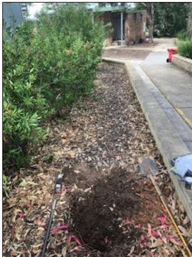
Image 38: Test pit HA03 (taken 13/04/2023)
