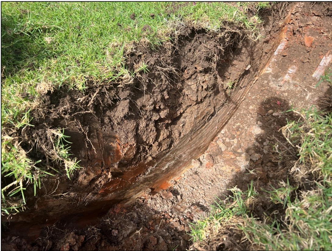
Image 24: Test pit TP08 (taken 13/04/2023)
