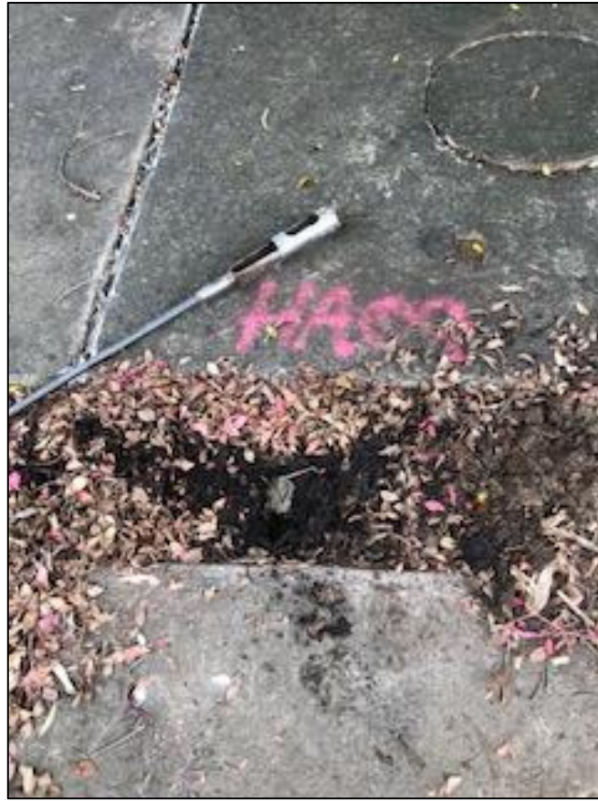
Image 41: Test pit HA09 (taken 13/04/2023)
