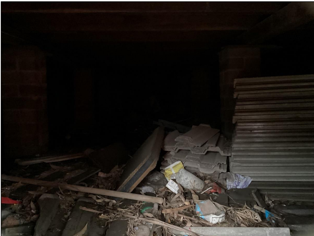
Image 6: General demolition waste and building materials observed within crawl spaces beneath buildings (taken 05/07/2022)
