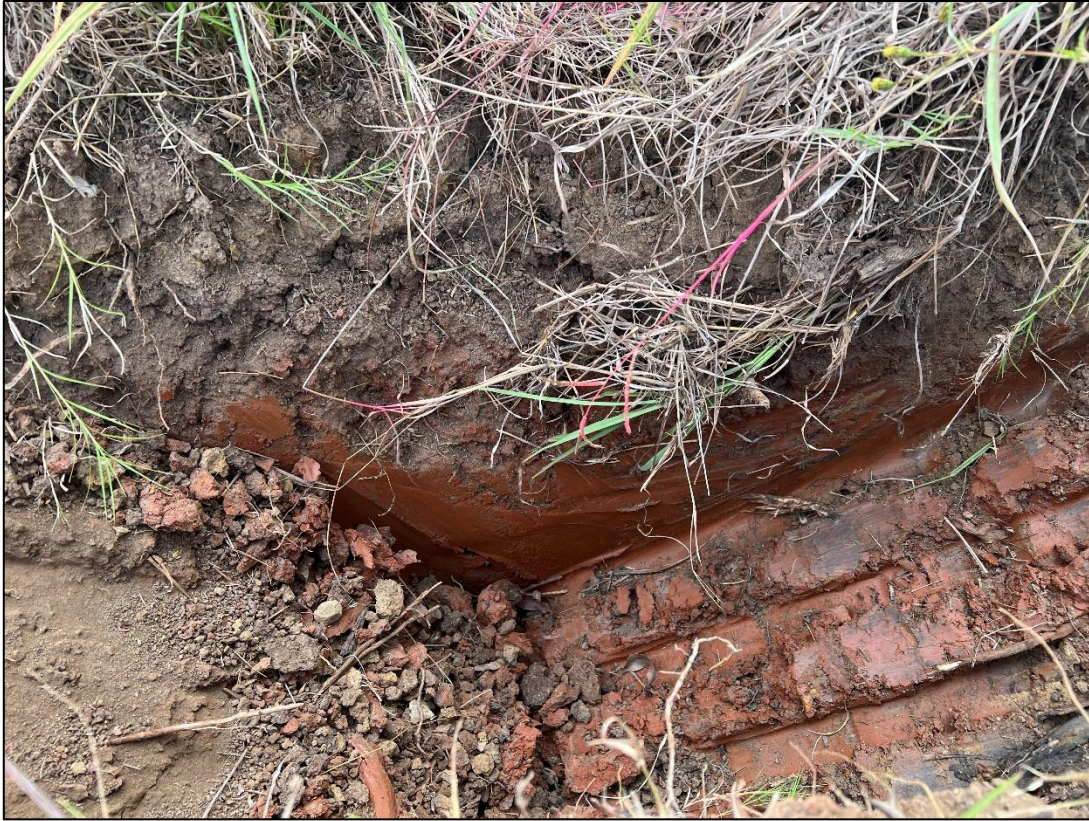
Image 17: Test pit TP02 (taken 13/04/2023)
