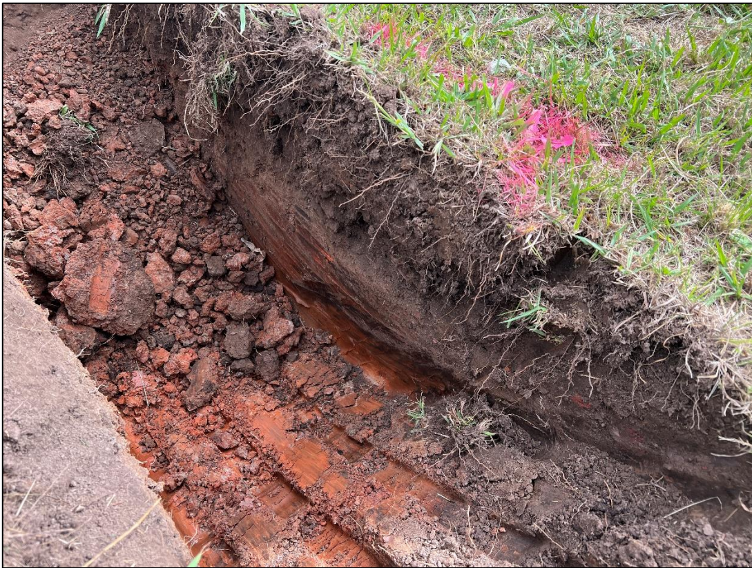
Image 20: Test pit TP04 (taken 13/04/2023)
