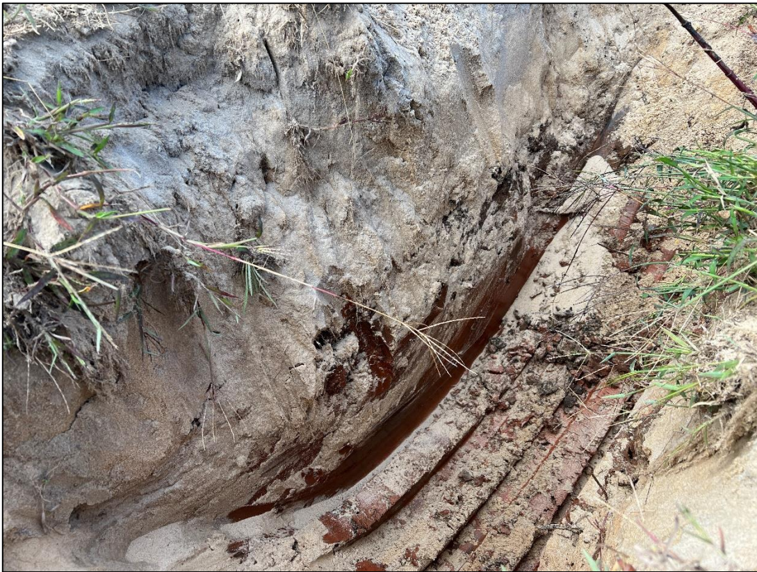
Image 28: Test pit TP14 (taken 13/04/2023)
